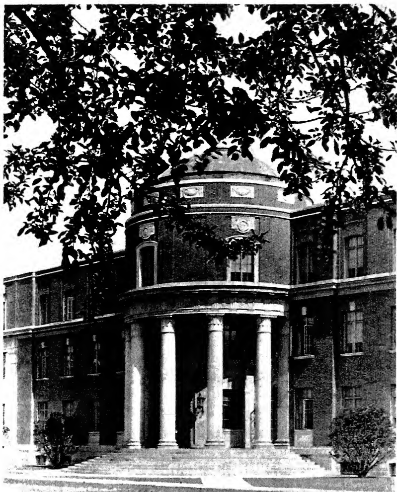
THE MINERAL INDUSTRIES BUILDING
